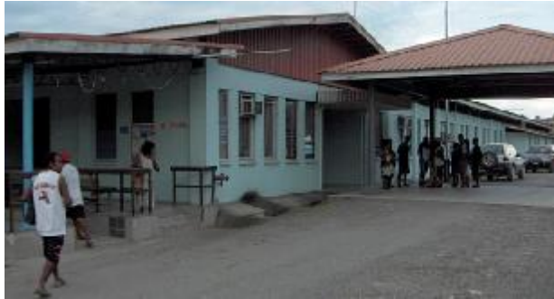
Emergency Entrance NRH
